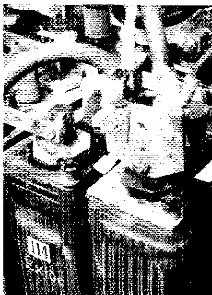
Part of the author's 12-V back-up power system, these 2-V, 300-Ah, lead-acid float cells—obtained free of charge from a local telephone company—help keep W4MLE on the air when commercial power fails. (W4MLE photos)
